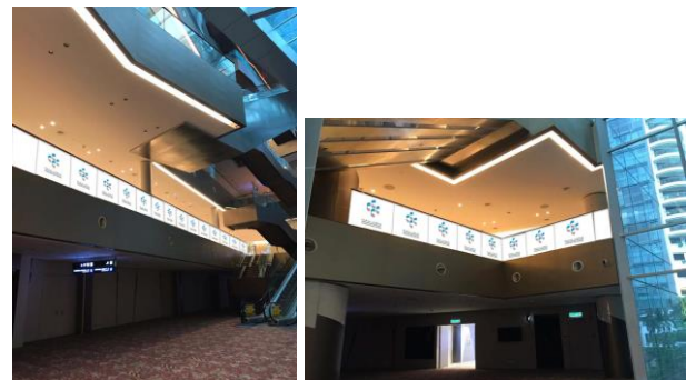
Glass Balustrade at Hall 6 Mezzanine Atrium Foyer
