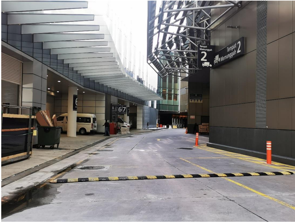
Drop off at loading bay 2 to enter Exhibition Hall 2
