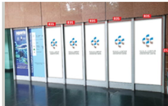
Exterior Facade Glass Wall (West Wing) GF002
