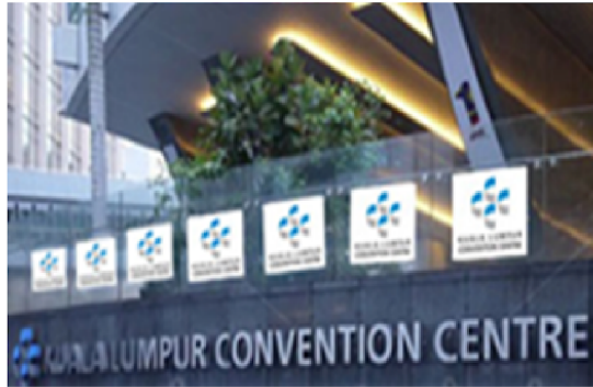
Glass Balustrade at the Water Feature ME001
